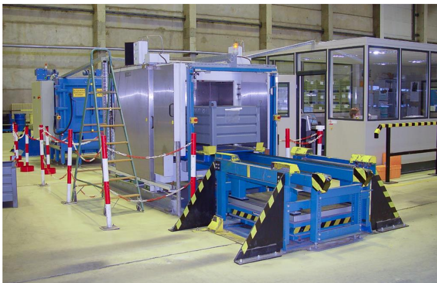
Figure 11: Decision measurement of components in the clearance measurement facility with detectors installed at all sides (EWN Entsorgungswerk für Nuklearanlagen GmbH, Greifswald nuclear power plant)
