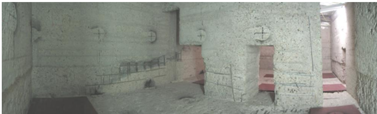
Figure 4: Decontaminated building structures (PreussenElektra GmbH, Kernkraftwerk Würgassen)
