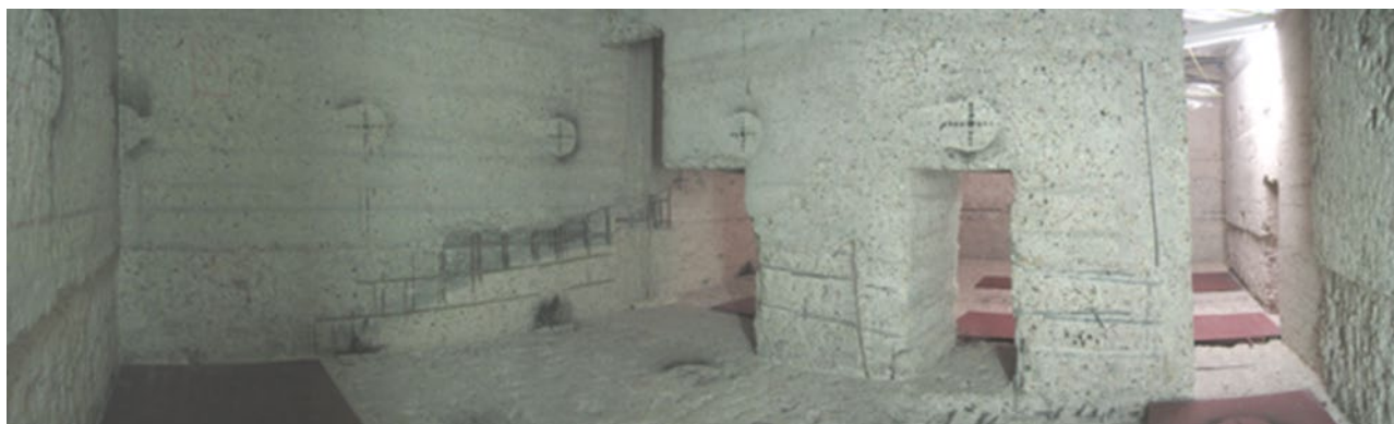
Figure 4: Decontaminated building structures (PreussenElektra GmbH, Würgassen nuclear power plant)
